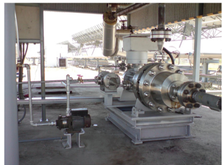
Hermetic Canned Motor Pump in operation in Spain at the Plataforma Solar de Almeria (PSA), pumping water 300°C with 100bar system pressure (Image courtesy of Auquime SA)
